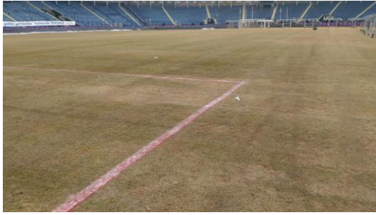
Pitch without under-soil heating – unable to produce adequate grass cover for a UEFA match.
