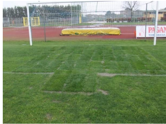
Poor surface levels in a re-turfed goal mouth.
