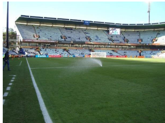
Irrigation system with low sprinkler pressure – leads to poor irrigation coverage.
