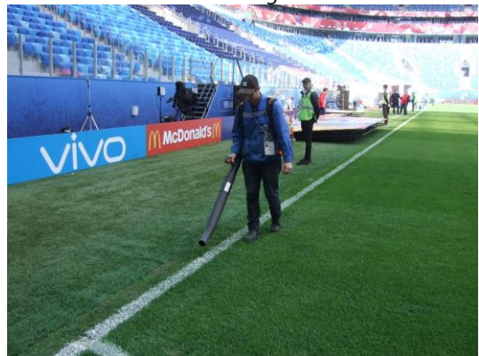
Wet paint – accelerate the drying of line marking using a leaf blower.
