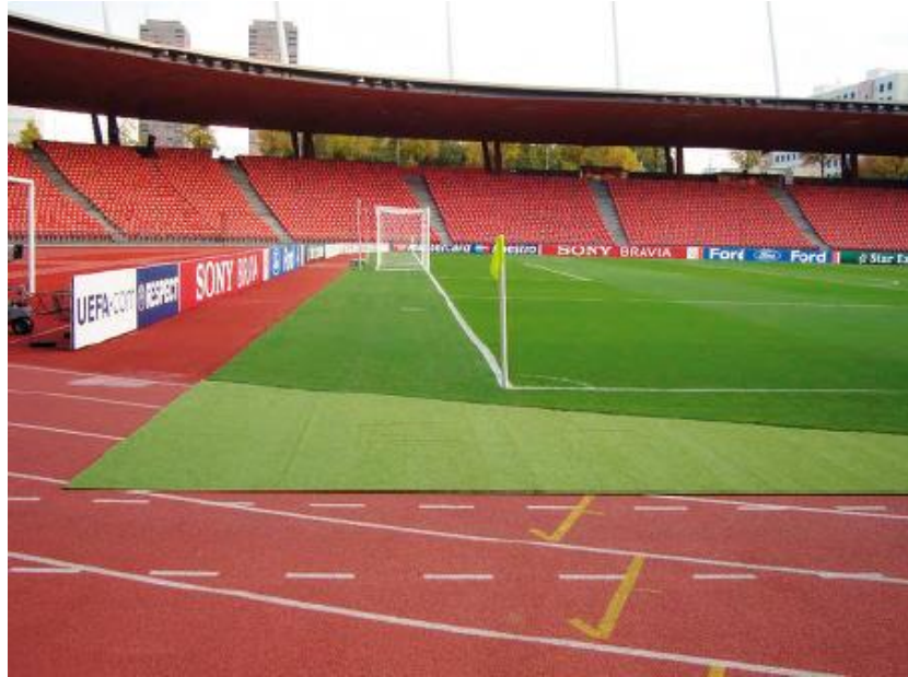
Fig. 27. Extension of turf perimeter around the field of play using high-quality artificial turf.
