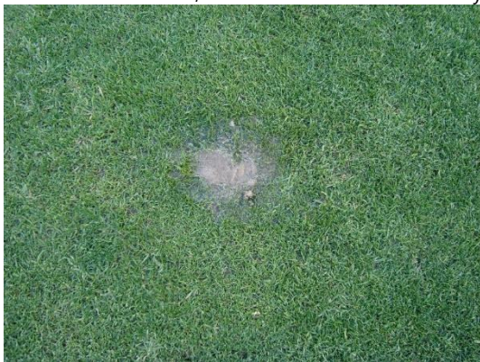
Leaking irrigation sprinkler head – if not repaired, surface damage will be extensive.
